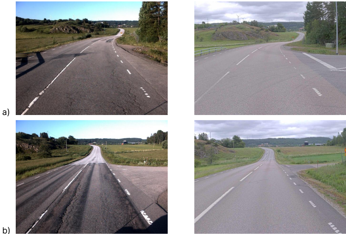
Figure 1. Photos from road 174 a) close to the bridge over the E6 and b) a little bit further down the slope. The left photos are taken in 2017 before the maintenance work and the right photos are taken in 2022, four years after the maintenance work. Photos: Trafikverket, PMSv4.
